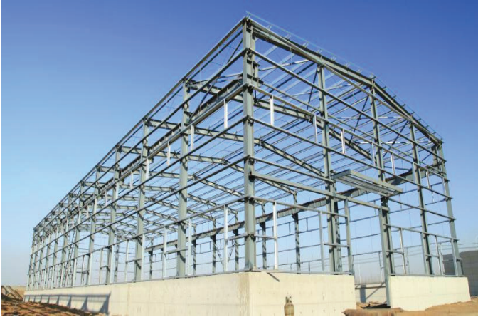
Structural Steel works for godowns and factory sheds
