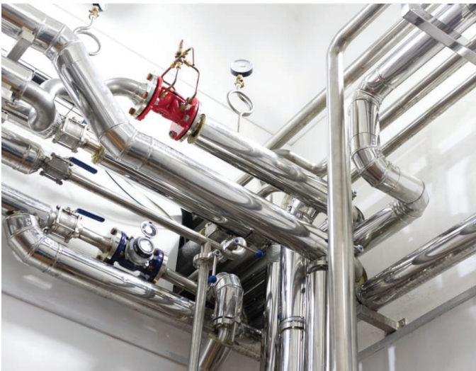
Supply and installation of steam piping
