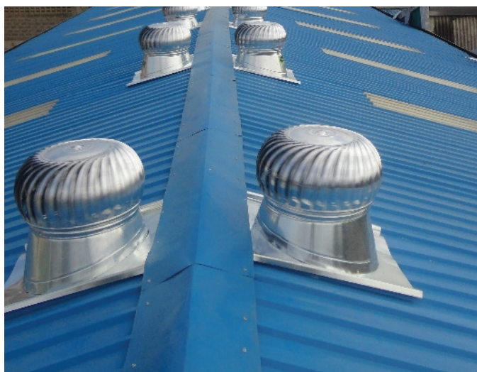
Roof Cyclone Ventilators
